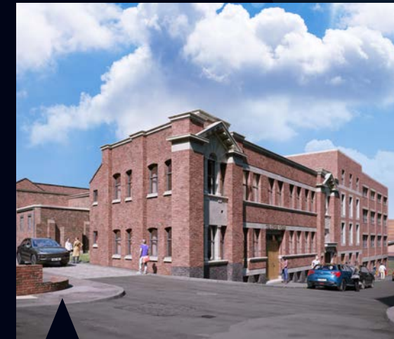
THE COPPERWORKS Birmingham
