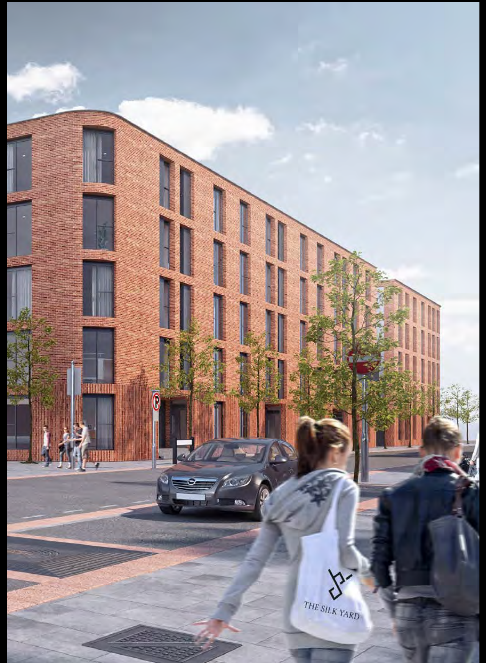
EXTERIOR VIEW, CASTLEWARD BOULEVARD
